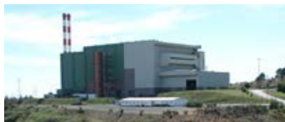
Osmose Inversa (10m³/h)
